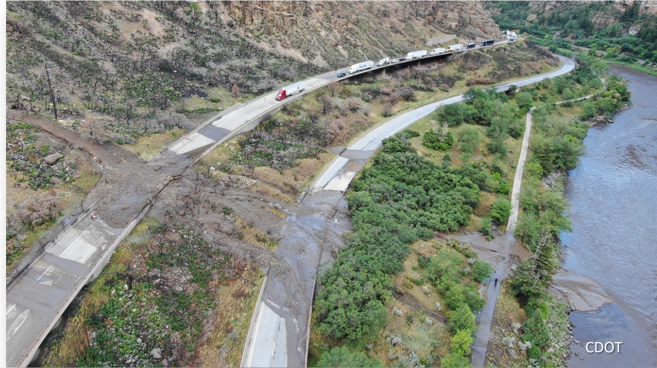
Interstate 70 through Glenwood Canyon, Colorado has been under threat to debris flows for several years since the 2020 Grizzly Creek Fire
